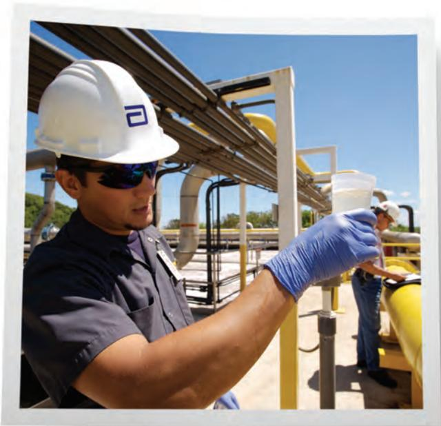
At our state-of-the-art biologics plant in Barceloneta, Puerto Rico, Richard Garcia, an environmental technician, checks a water sample at a stage one station. The plant processes its waste water in three stages before sending it to the municipal waste water treatment plant.
