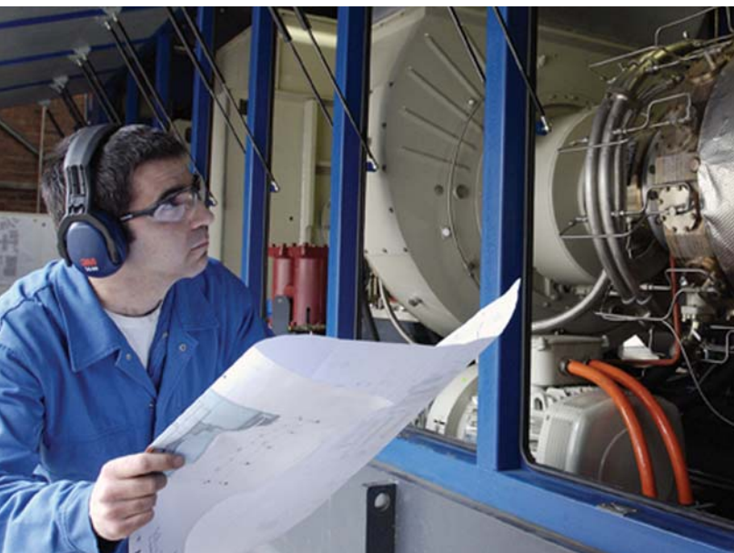
Claudio Monni, a mechanic and boilerman at Abbott Germany in Ludwigshafen, checks the installation of a cogeneration unit.
